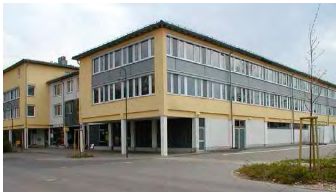
Allectra GmbH facility near Berlin (Germany)
